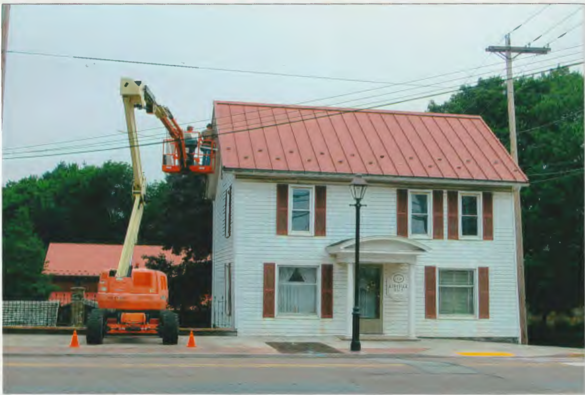
DON WILAND, CONTRACTOR, WORKING ON THE INSTALLATION OF SOFFIT AND FASCIA ON THE HERITAGE HAUS. JULY 21, 2022.
